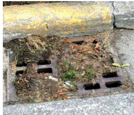
Residents can help make the system work more efficiently by making sure the openings are clear of debris and trash. This is the first step in allowing stormwater to enter the system and is an easy way to help prevent flooding at a local level.
