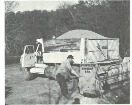
Spreading Road Slag
