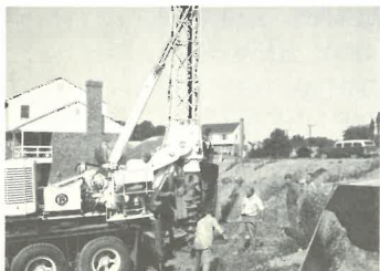
Drilling for piers to solid ground
